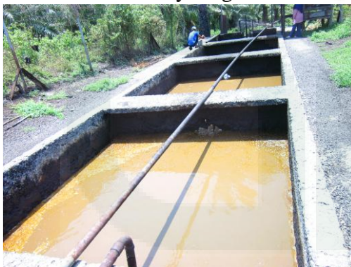
Gambar 13. Kolam Sludge fit
