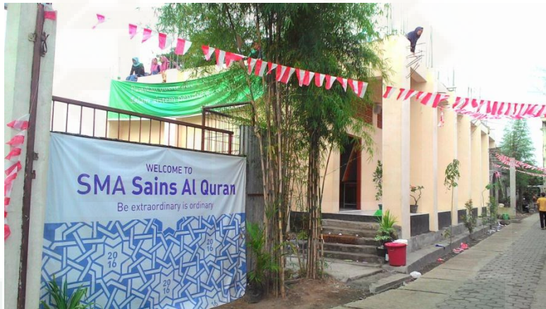
Gedung SMA Sains Al-quran
