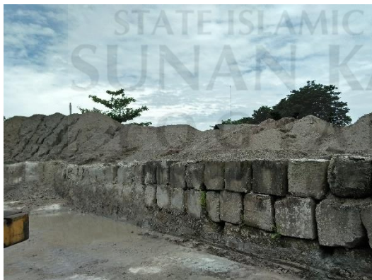
Stock Pile Material
