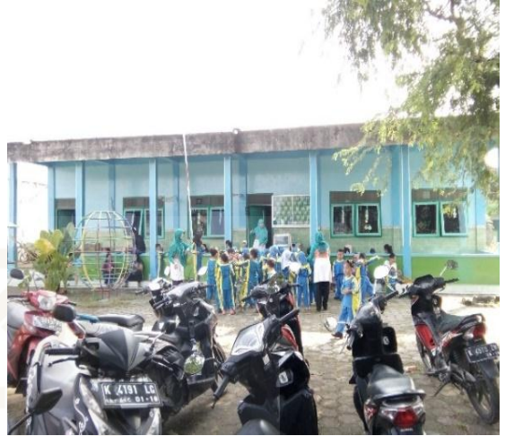
TK Ar-Rohman tampak depan
