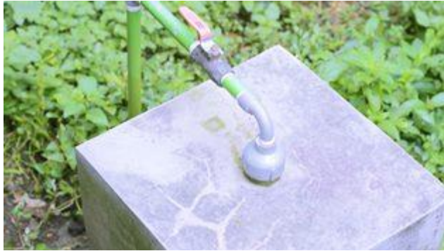
Gambar 4. Kran biogas
